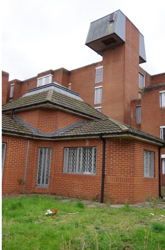
Figure 1.15: Existing buildings within the prison
