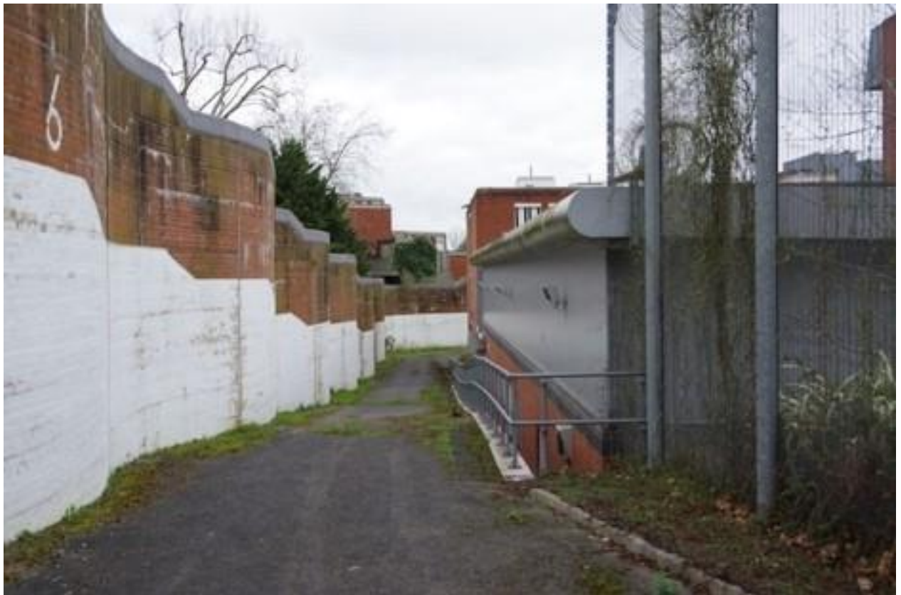
Figure 1.12: Looking NE to Bakerfield Estate (within wall)
