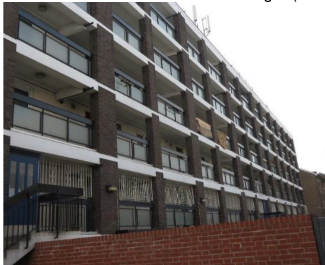
Kimble House elevation facing the site, showing the overhanging walkways
