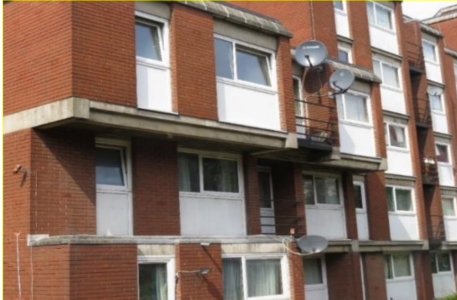
Neighbouring Bakersfield Estate elevation, showing the architecture causes overhangs to a number of windows
